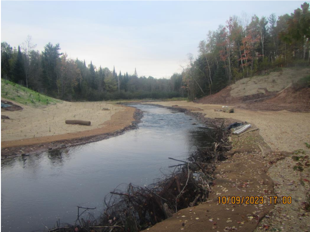
Facing upstream from where culvert and railroad grade was removed
