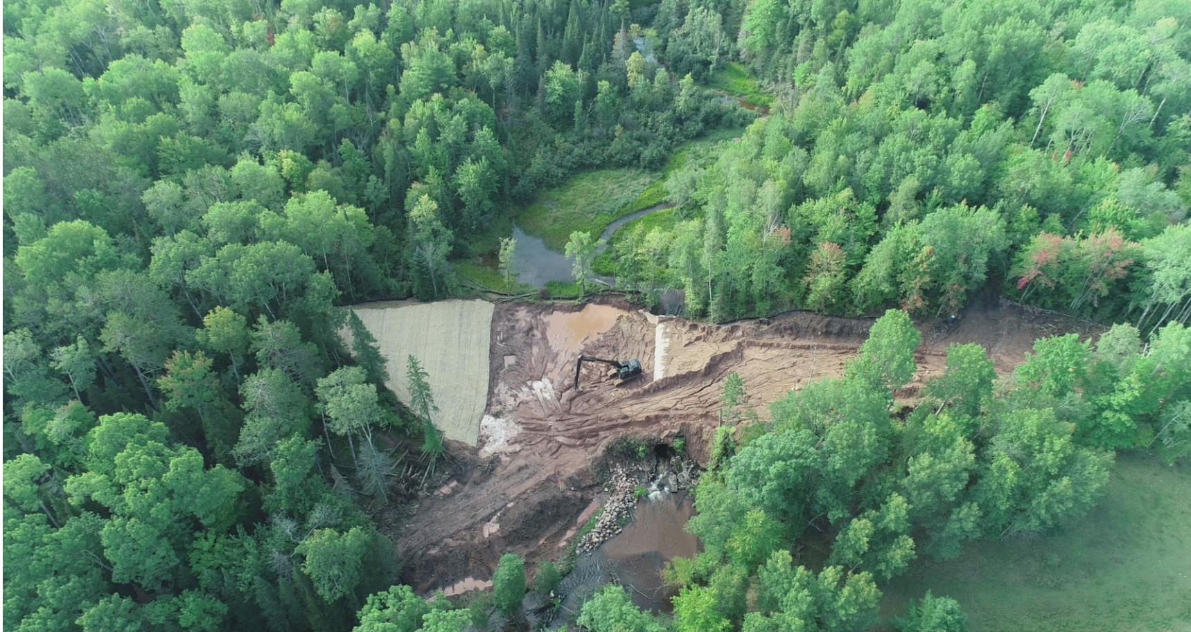
Aerial view of railroad grade and culvert removal September 2023
