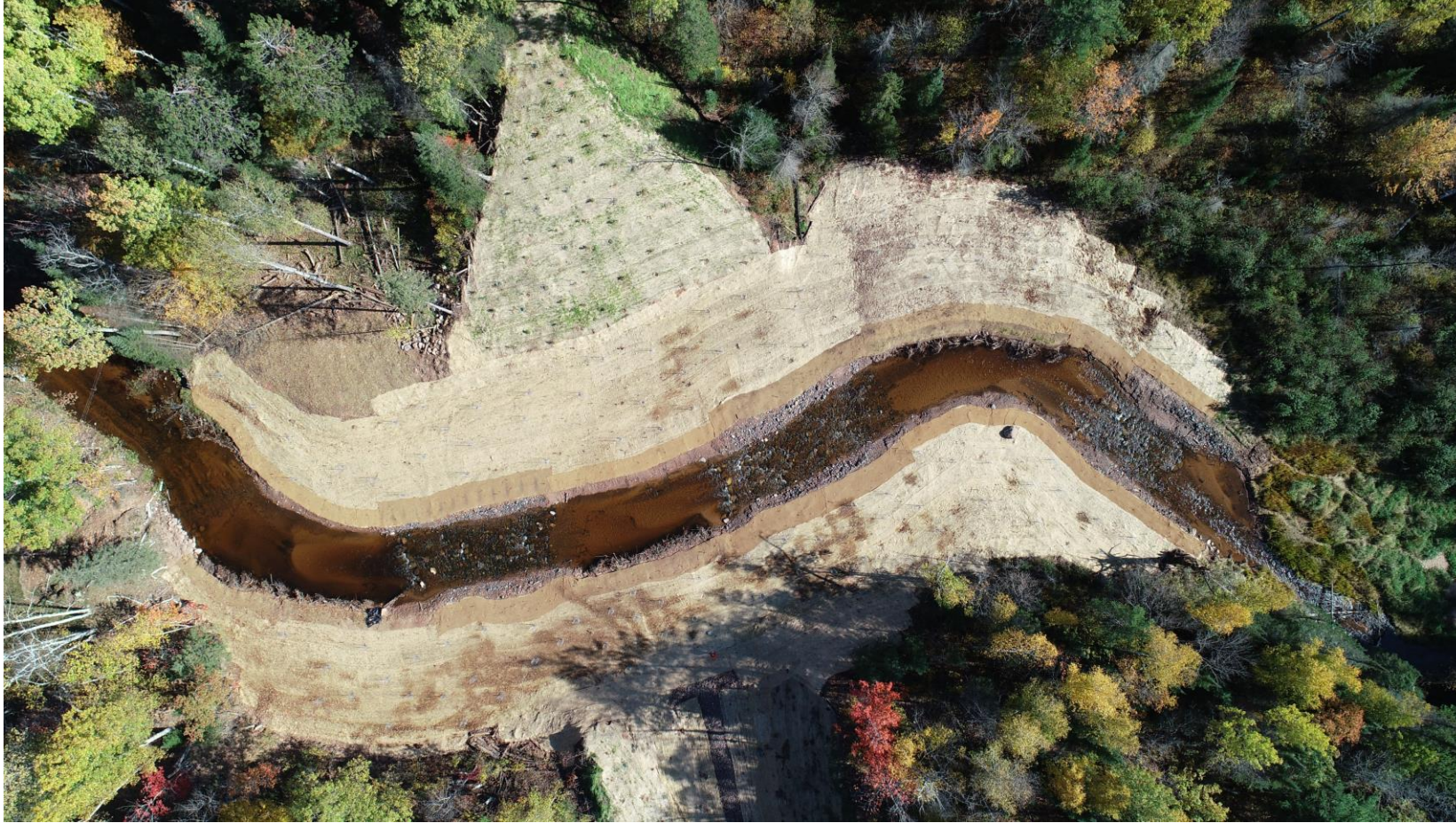
Aerial view of new channel October 2023
