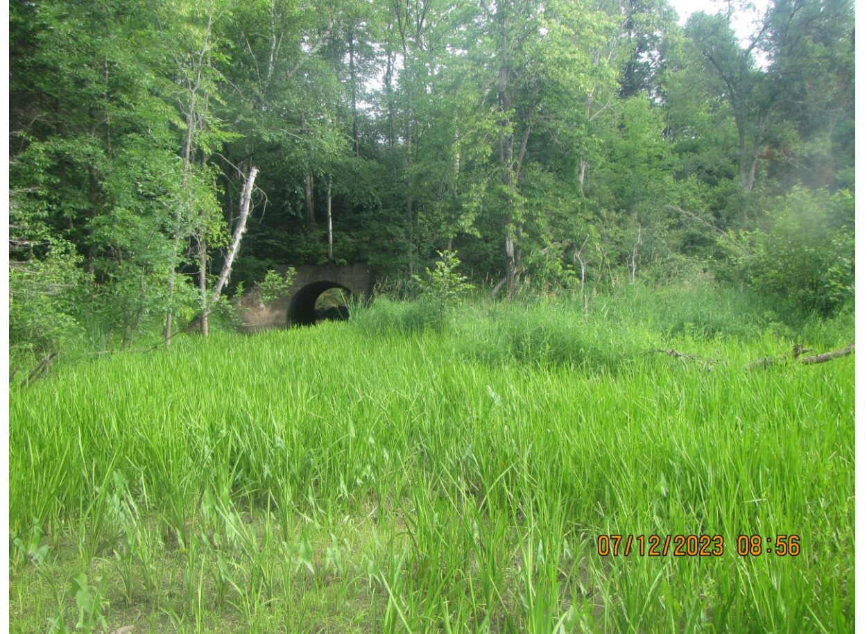
Upstream of culvert July 2023
